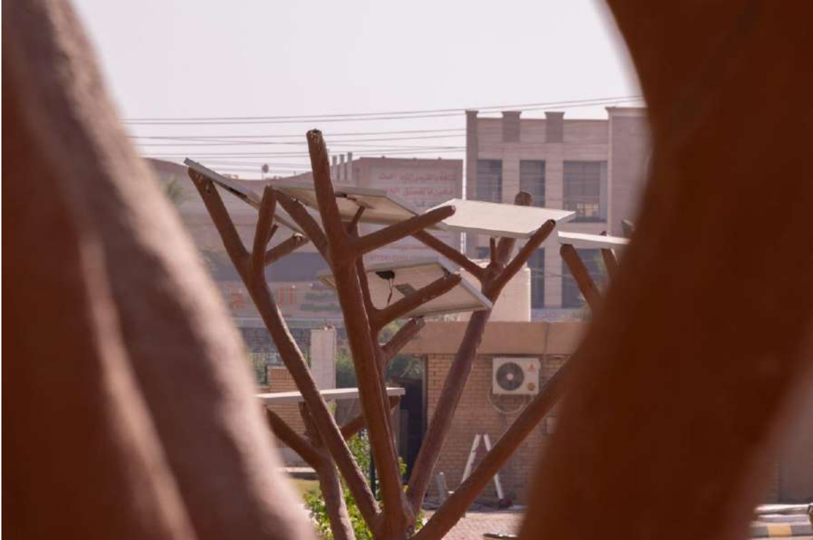
Decorative trees with solar panels
